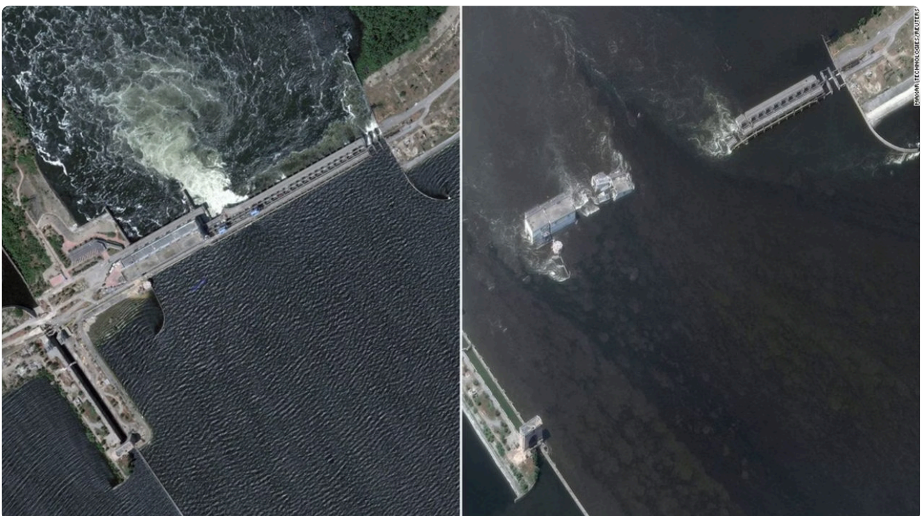
Before and after satellite images of Nova Kakhovka dam. Source: UWEC, 2023.
